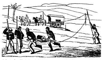
A drawing from Myer's *Manual of Signals* illustrating the field, or flying, telegraph. It shows the wagon with batteries and instruments. The wire (in this case presumably bare copper, since it is being strung on insulators on poles) is being run out from a reel carried by two men. The linesmen are using a crowbar to open holes to receive the lance poles. Myer estimated that  $2\frac{1}{2}$  miles of such wire line could be put up in an hour.
