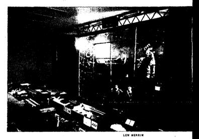
In radar control center today, mass of data is written backward on transparent board so the officers in front can read it. This method clumsy, complicated and (due to confusion) potentially dangerous—has been made obsolete by development of a new electronic computer
